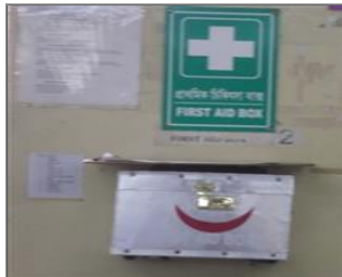
Photo first aid facilities C2 First Aid Facility.jpg
